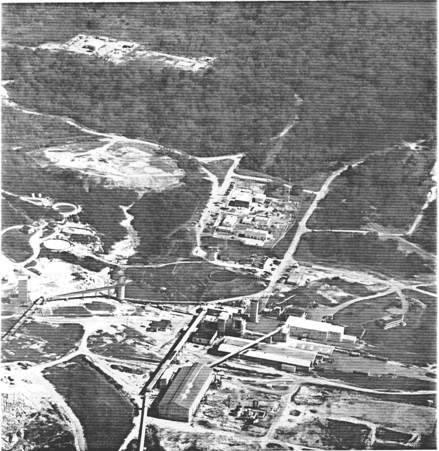
WEST HATCHERY Figure 1-7. Weeks Island SPR Site The West Hatchery (WH) site is located in Cameron Parish, 29 km (18 mi) northwest of Lake Charles, Louisiana and 22 km (14 mi)
